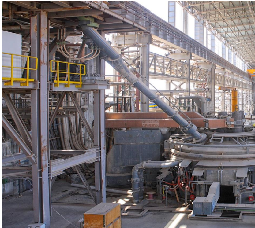
Fig. 7: DRI feeding pipe into EAF roof.
