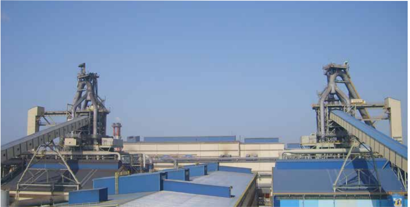
Dragon Steel Corporation, Taichung Blast Furnace No.1 and No.2
